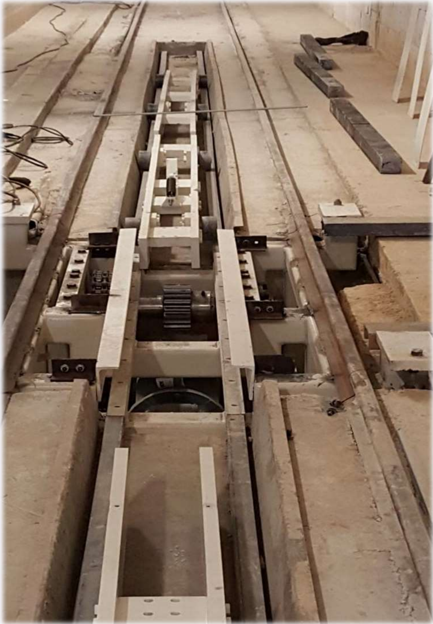
Pusher-Assembly- Istanbul Çatalca Ytong
