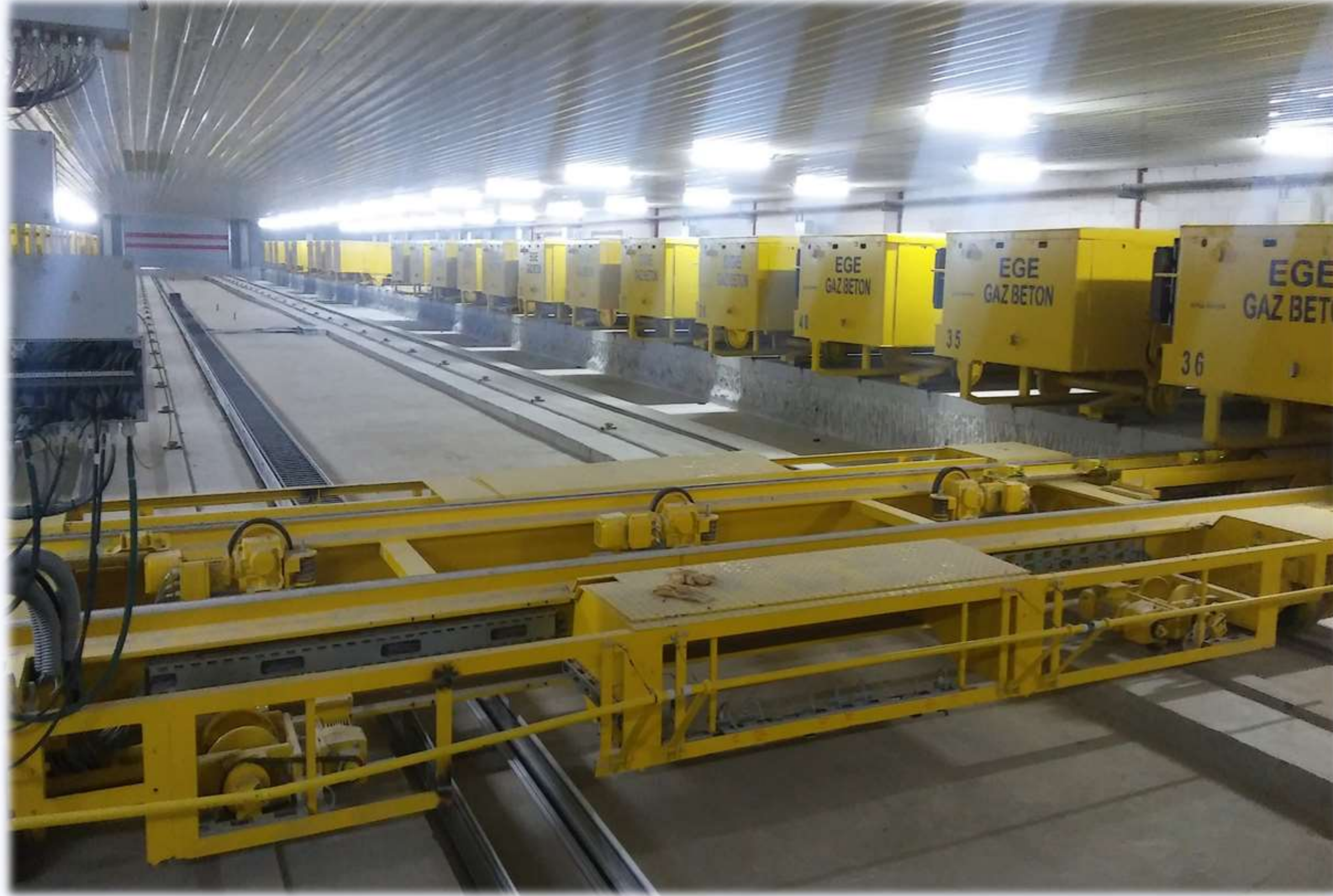
Fermentation Plant – Ege Gaz Beton Aydın Söke (Masa Project)
