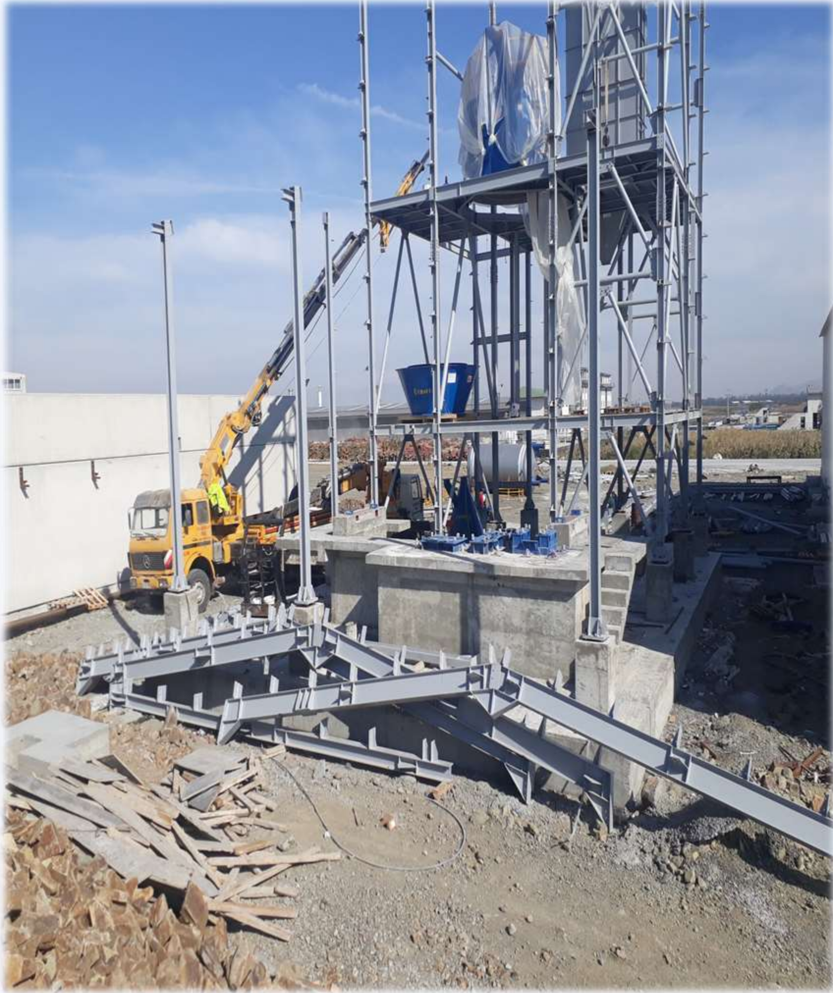
Lime Preparing Tower Plant Assembly- KÇS Aydın Söke
