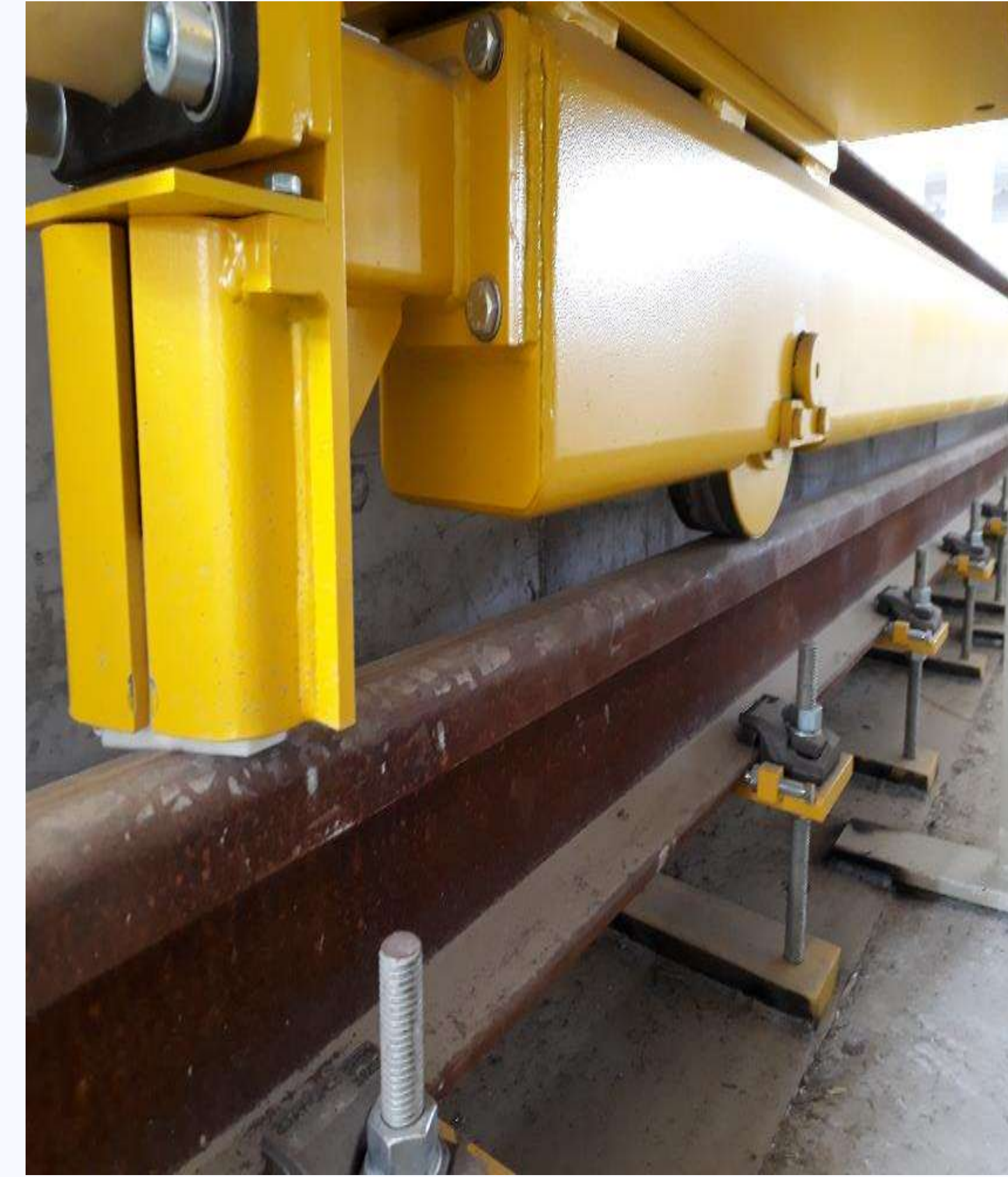
Cutting Line Assembly-KÇS Aydın Söke
