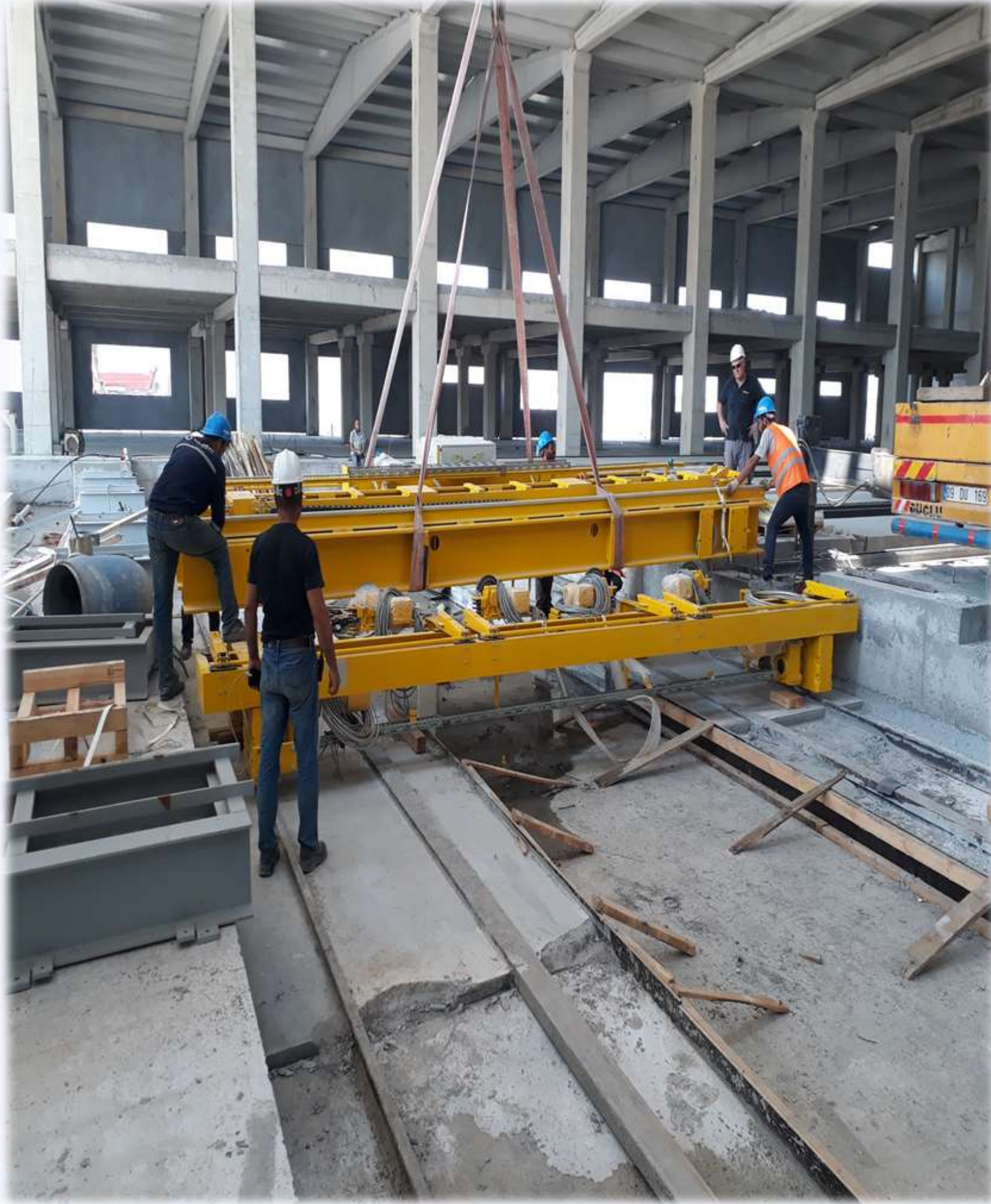
Autoclave Ground Crane Assembly- KÇS Aydın Söke
