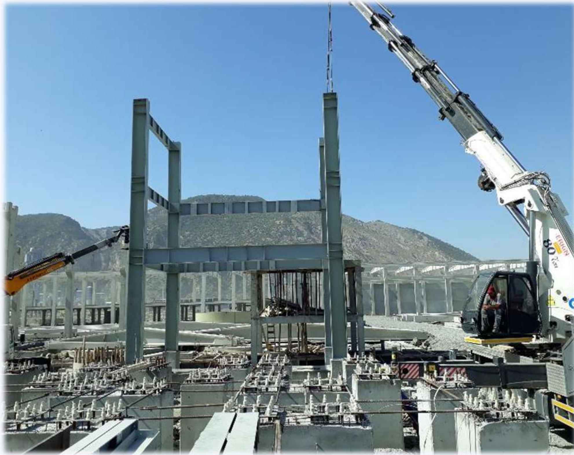
Mixing Tower Assembly-Aydın Söke KÇS (Masa Project)
