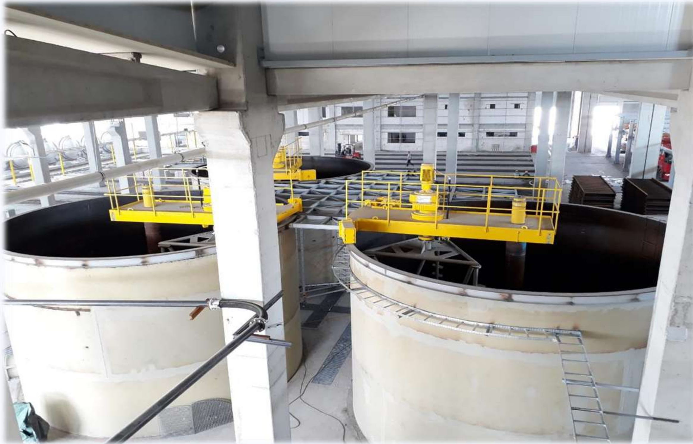
Sludge Tanks Manufacturing and Assembly – KÇS Aydın Söke (Masa Project)
